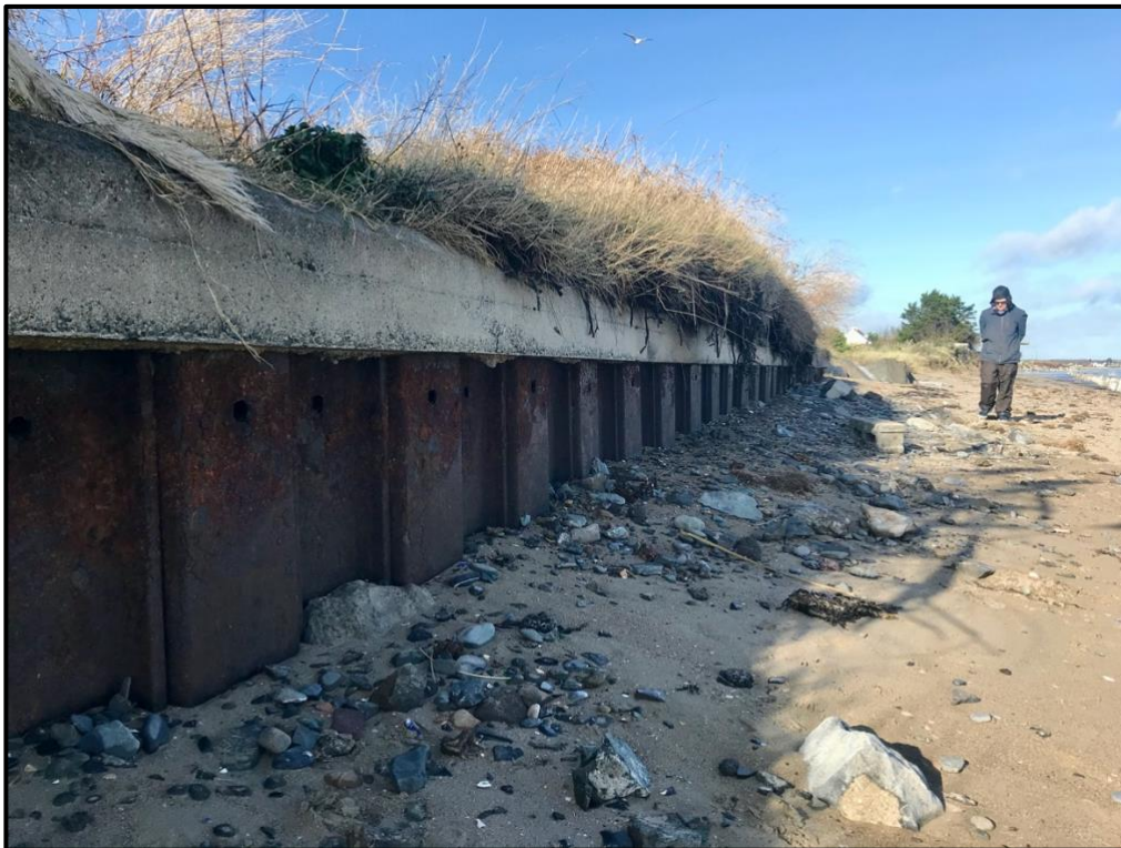
Figure 18: Evidence of the 1950s sheet pile located along the southern section of Burrow Beach.
