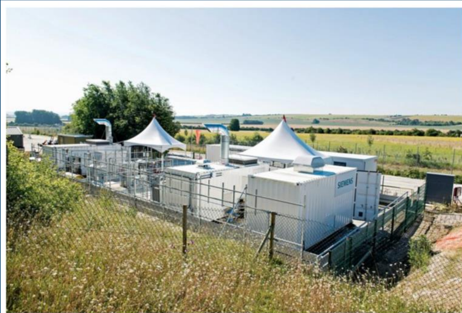
Figure 5.2. Green Ammonia Production System, from (Boerner, 2019)
